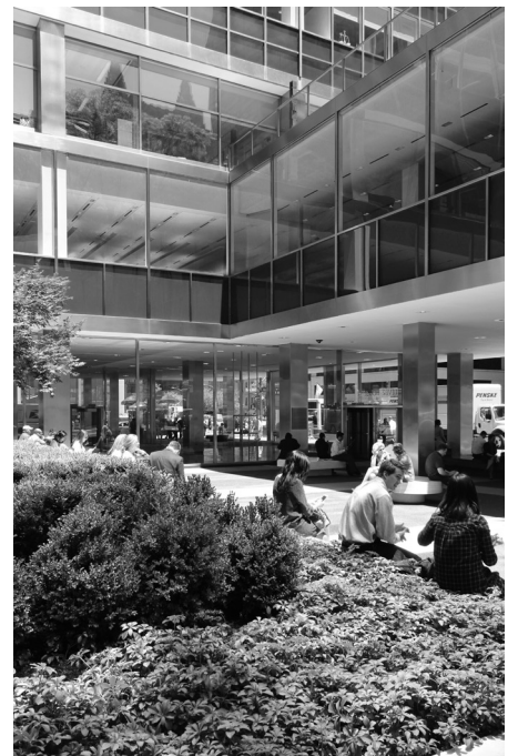
Figura 3. Lever House Building. Junio, 2016.
